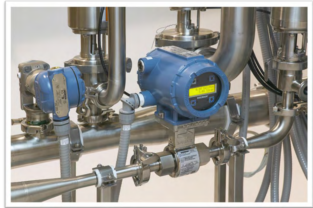
Flow meter installation
