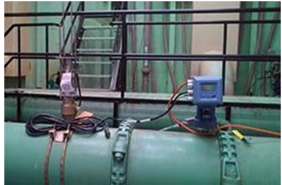
Use of electromagnetic flow meter to track water use in a rural area for allocation and conservation purposes.
