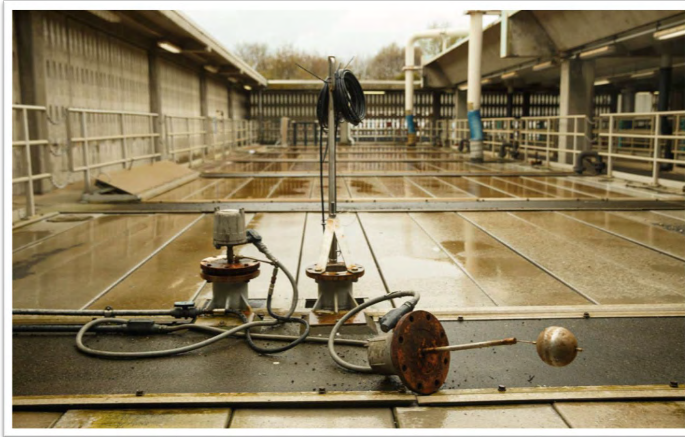
Failed float from West Point Treatment Plant
