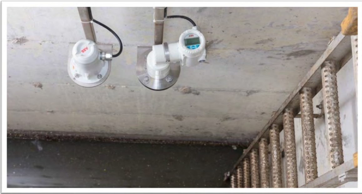
Laser sensors in a municipal well
